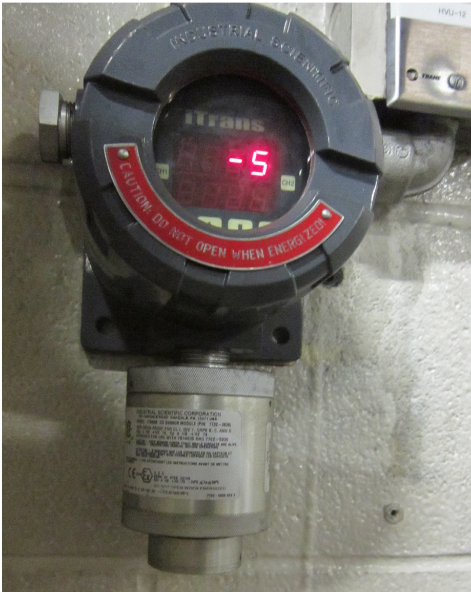
A gas detection system commonly monitors for methane, carbon monoxide and nitrogen dioxide in a CNG maintenance garage. A remote gas detector is shown above.
