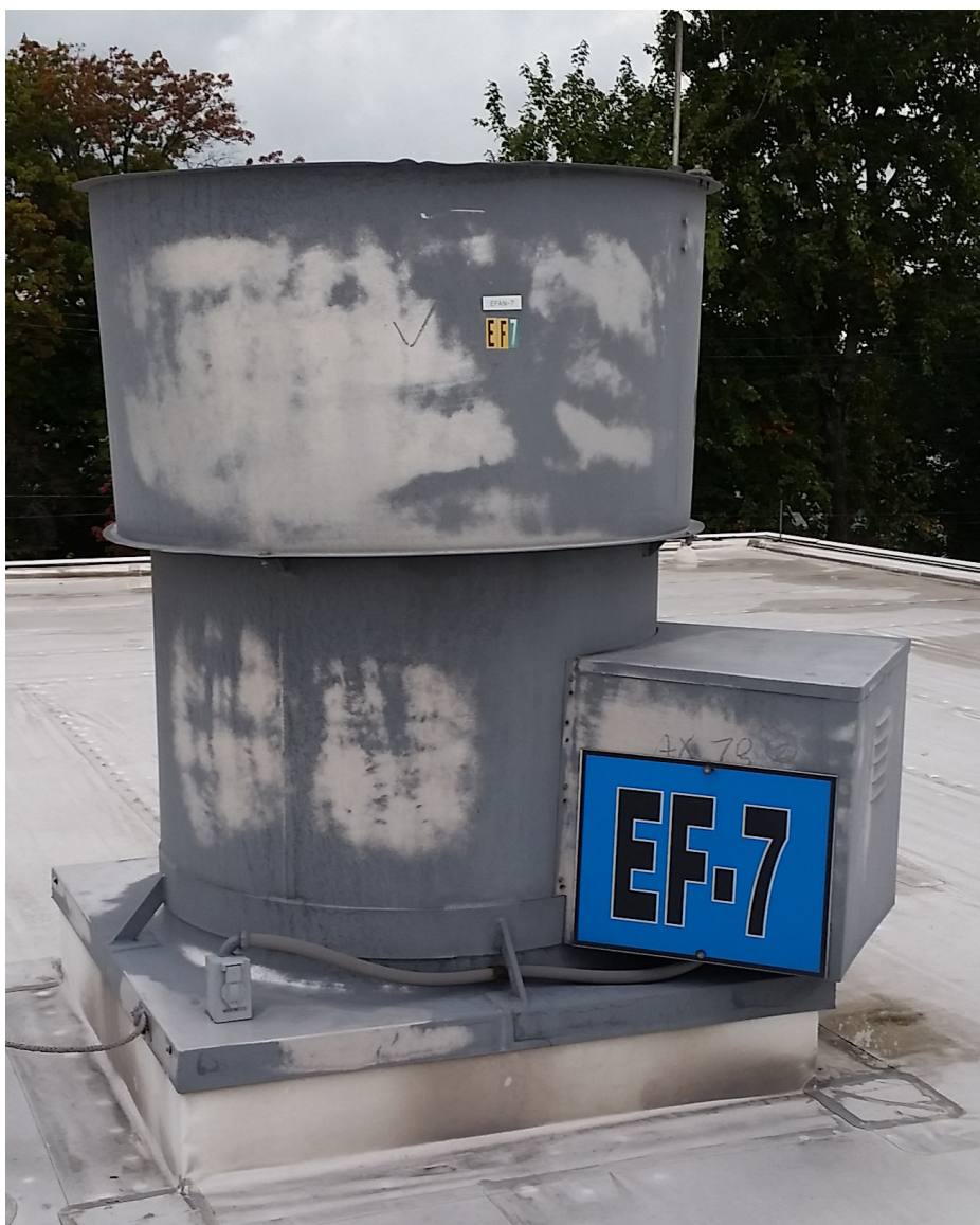
An emergency exhaust fan was installed on the roof of a major maintenance garage. It is interlocked with a methane detection system to purge the space if a methane leak is detected.
