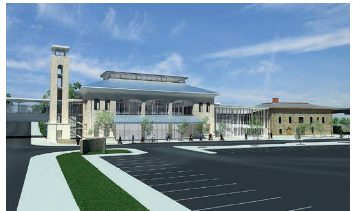
This Niagara Falls intermodal station is designed to be a focal point and impetus for tourism.
